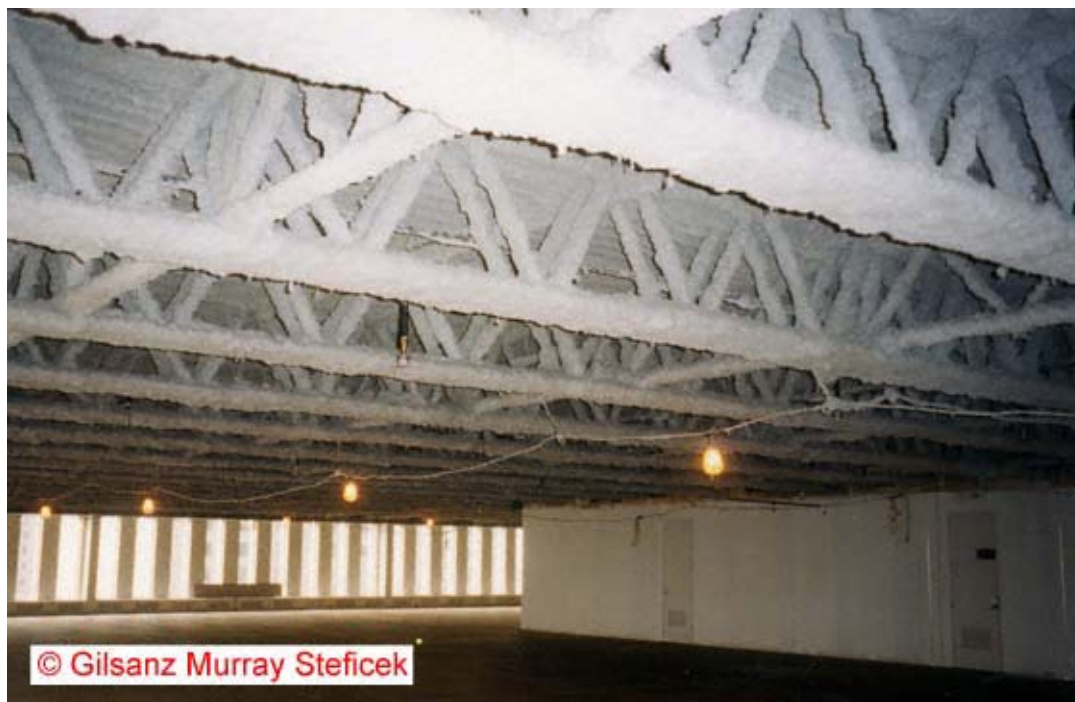
Figure 1–8. Photograph of insulated WTC trusses.
